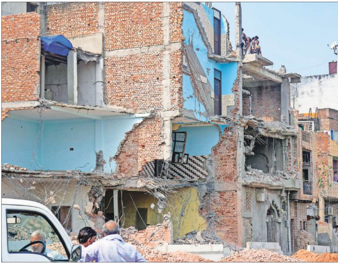
Demolished structures at the site following a demolition drive carried out by Civic Authorities on Max Hospital Road as part of a road-widening project, in New Delhi, on Wednesday. (PTI)
