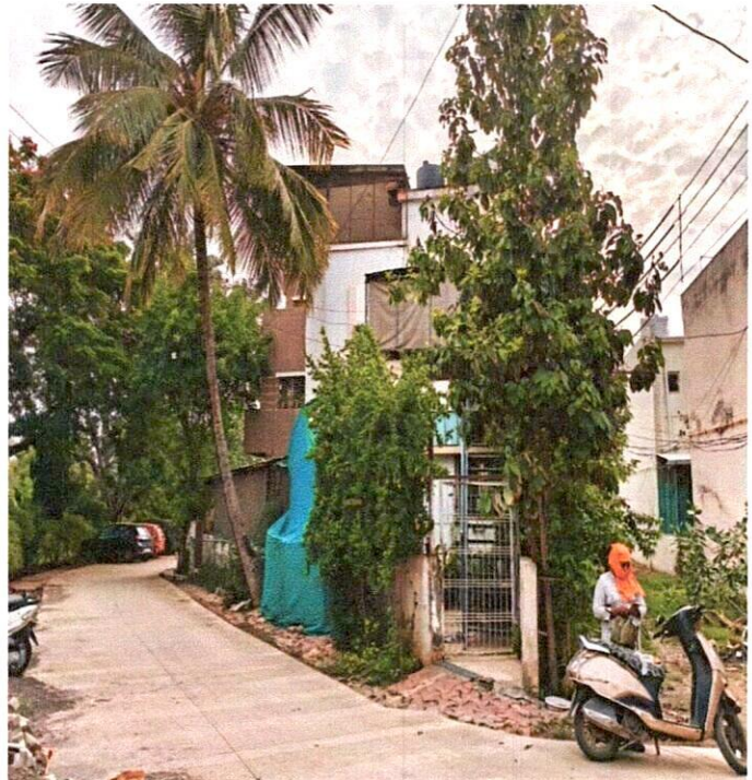
Roadside View of The Property
